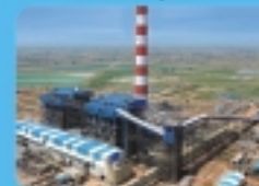
Rajapur Thermal Power Plant
